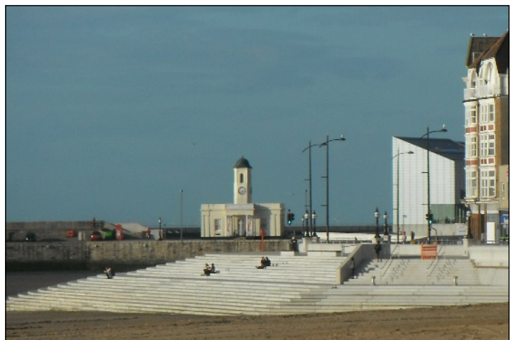
The Steps (Flood Prevention Works), Marine Drive, Margate
