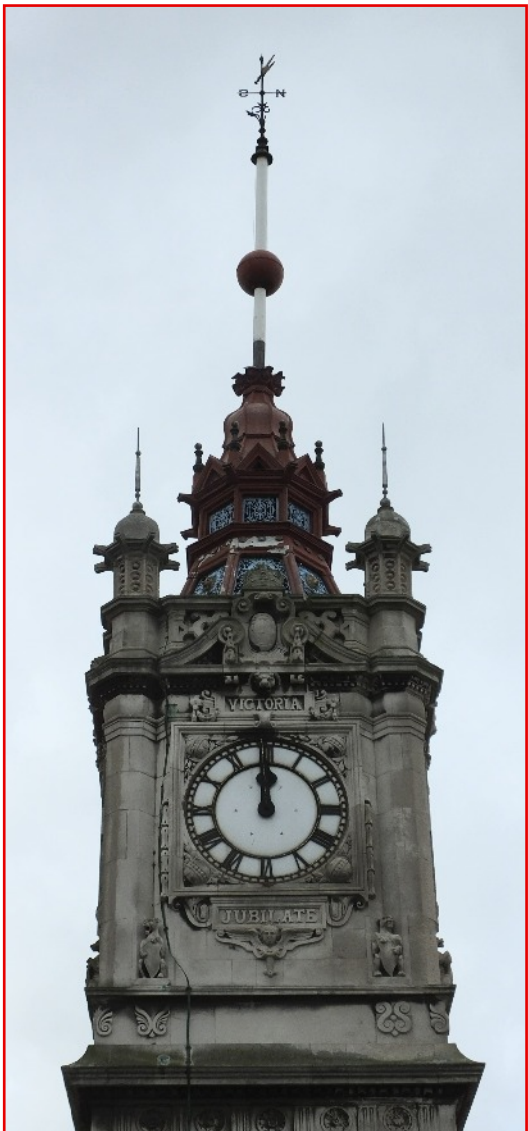
The hands on the Clock Tower clock point to the Time Ball halfway up the pole at mid-day on 16th January
