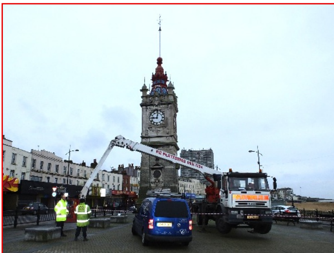
Work starts promptly at 9.00am on 16th January 2014
